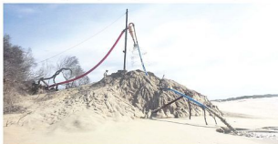
Dredging sand onto the most vulnerable areas of the 'Spit' dune, which separates St Francis Bay's canals from the sea.
