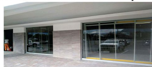
Pro Glass installation at a most recent shopfront
